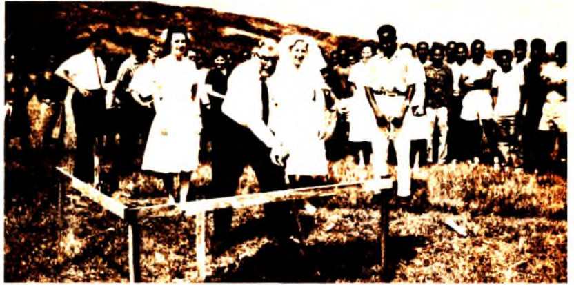
General Superintendent Samuel Young breaks ground for the new Nazarene hospital in New Guinea. The nurses in the foreground are Mrs. Helen Bolerjack, left; and Mrs. Margaret Bromley, right. Construction of the hospital is being supervised by Mr. Kenneth Dodd of Newport, Oregon. Dr. and Mrs. Dudley Powers are scheduled to go to New Guinea this fall to have charge of the hospital. A denominational "special" of $213,000 is financing the construction.
