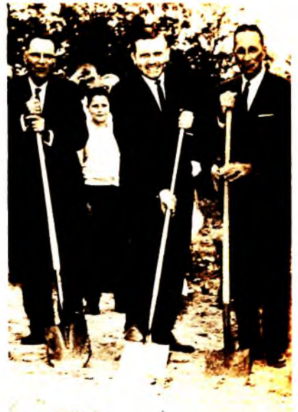
Ground breaking for the new, relocated First Church, Little Rock, Arkansas, drew two hundred people to the site at Evergreen and Mississippi Avenues. Participants in the ceremony, left to right, were Dr. A. Milton Smith, South Arkansas District superintendent; Rev. Thomas M. Hermon, pastor; and Richard Gates, of the Worthen Bank and Trust Company. About twelve months will be required for completion of the new structure, valued at $450,000.
