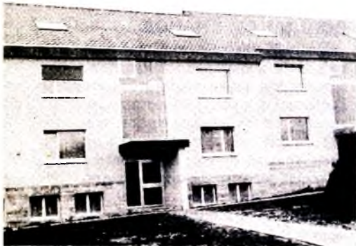
New dormitory at European Nazarene Bible College provides housing for staff members and married students.
