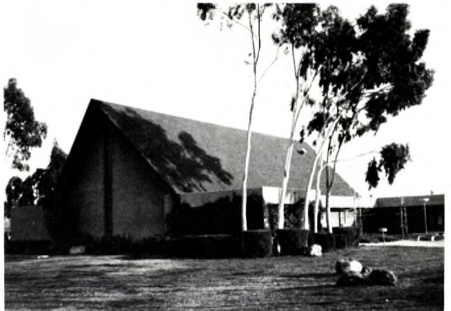
Present facility of the Glendora church
